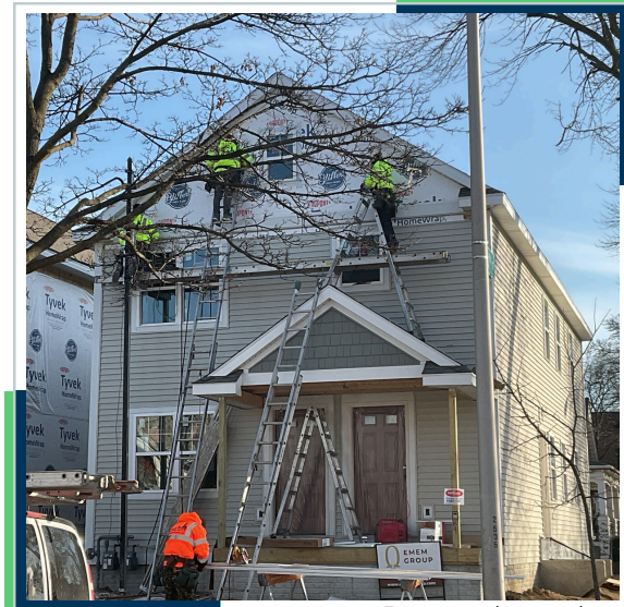
Emem workers at the Midtown Duplexes project.
